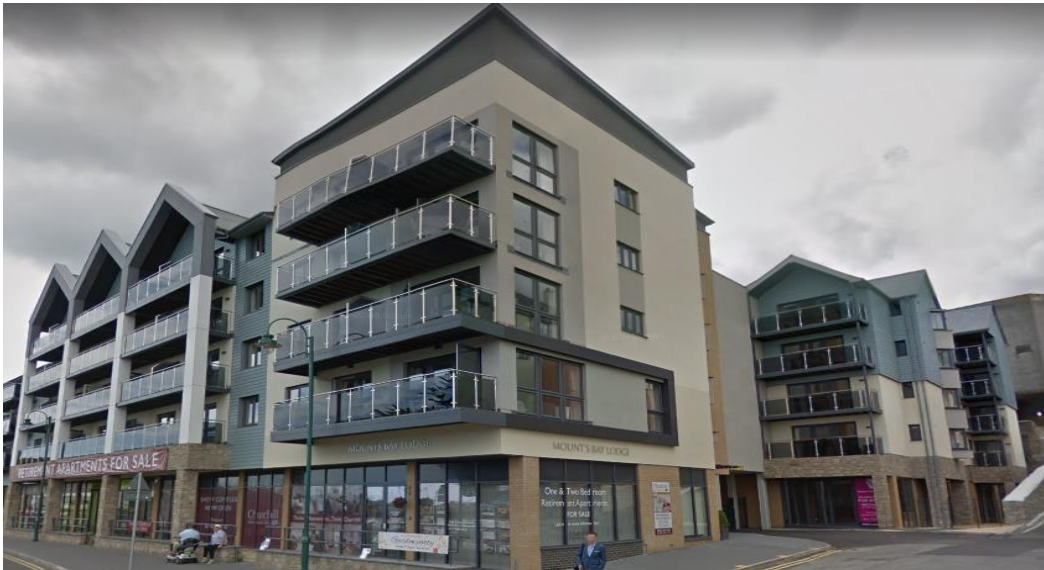
Mounts Bay Retail Centre - Completed 2018
