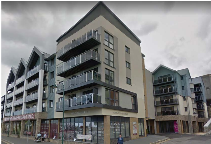
Mounts Bay Retail Centre - Completed 2018
